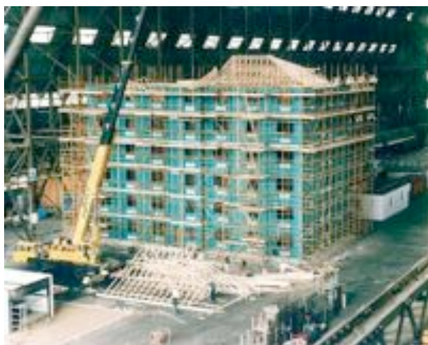
Figure 2: Timber Frame 2000. Platform timber frame incorporating engineered wood products. Image copyright TRADA
