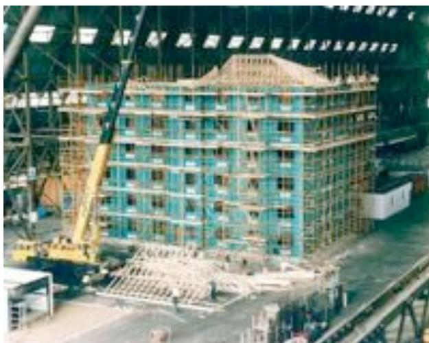
**Figure 2: Timber Frame 2000. Platform timber frame incorporating engineered wood products. Image copyright TRADA**
