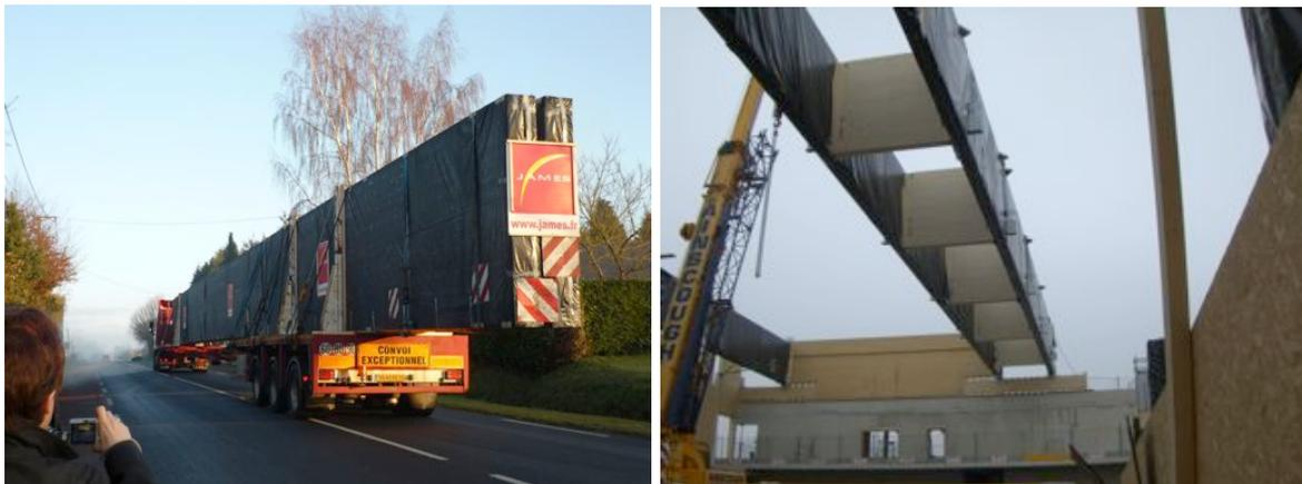
**Figure 10: Eton Manor sports facility. Delivery and installation of main beams. Image copyright PJ Steer.**
