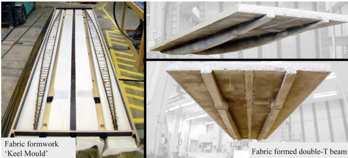
Figure 3. 4m span double T beam construction
