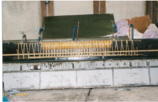
Figure 9. FRP helix being tied into reinforcing cage.
