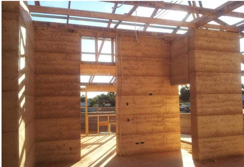
*Figure 6. Rammed earth is sustainable, cheap, simple to build with, but not very popular. Is its incompatibility with the typical construction processes of the informal sector part of the explanation? Unaltered image courtesy of Daniela Ciancio, via <http://theconversation.com/cheap-tough-and-green-why-arent-more-buildings-made-of-rammed-earth-38040> Licensed under Creative Commons CC BY-ND 4.0 <http://creativecommons.org/licenses/by-nd/4.0/legalcode>*
