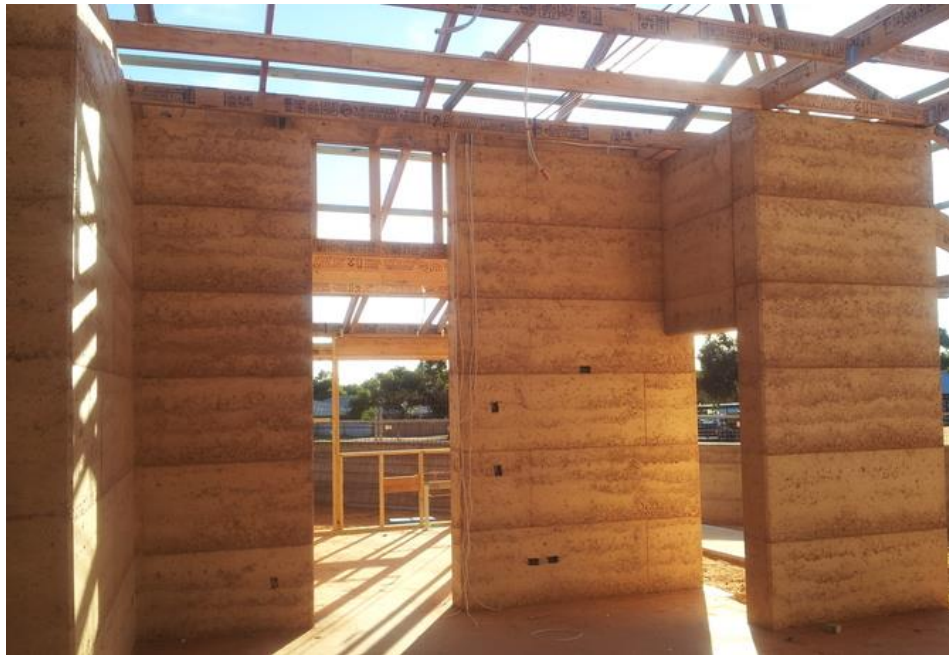
Figure 6. Rammed earth is sustainable, cheap, simple to build with, but not very popular. Is its incompatibility with the typical construction processes of the informal sector part of the explanation? Unaltered image courtesy of Daniela Ciancio, via http://theconversation.com/cheap-tough-and-green-why-arent-more-buildings-made-of-rammed-earth-38040 Licensed under Creative Commons CC BY-ND 4.0 http://creativecommons.org/licenses/by-nd/4.0/legalcode
