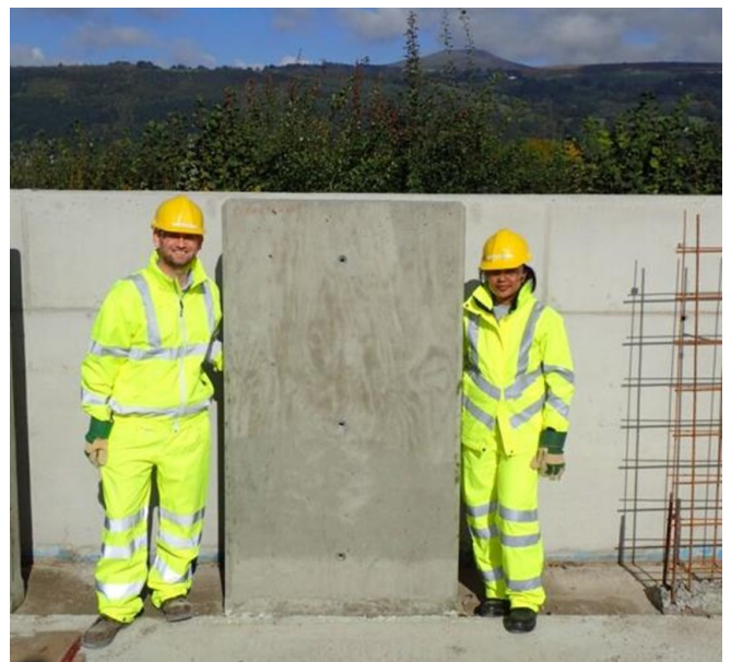
Figure 4: Finished wall with bacterial self-healing agents.
