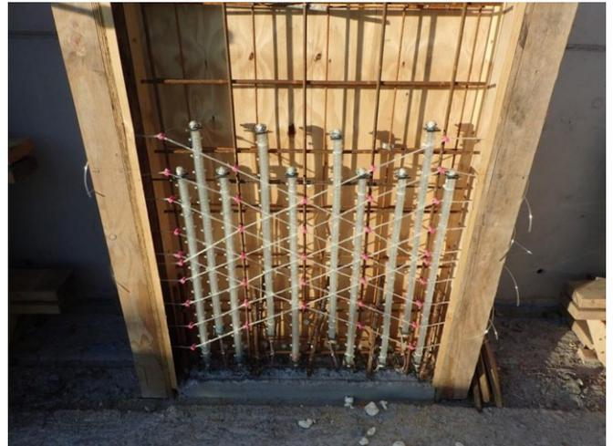
Figure 3: Shape memory polymers inserted at the base of a concrete wall (large vertical elements) and vascular network of tubes (diagonal elements) which will be removed after casting
