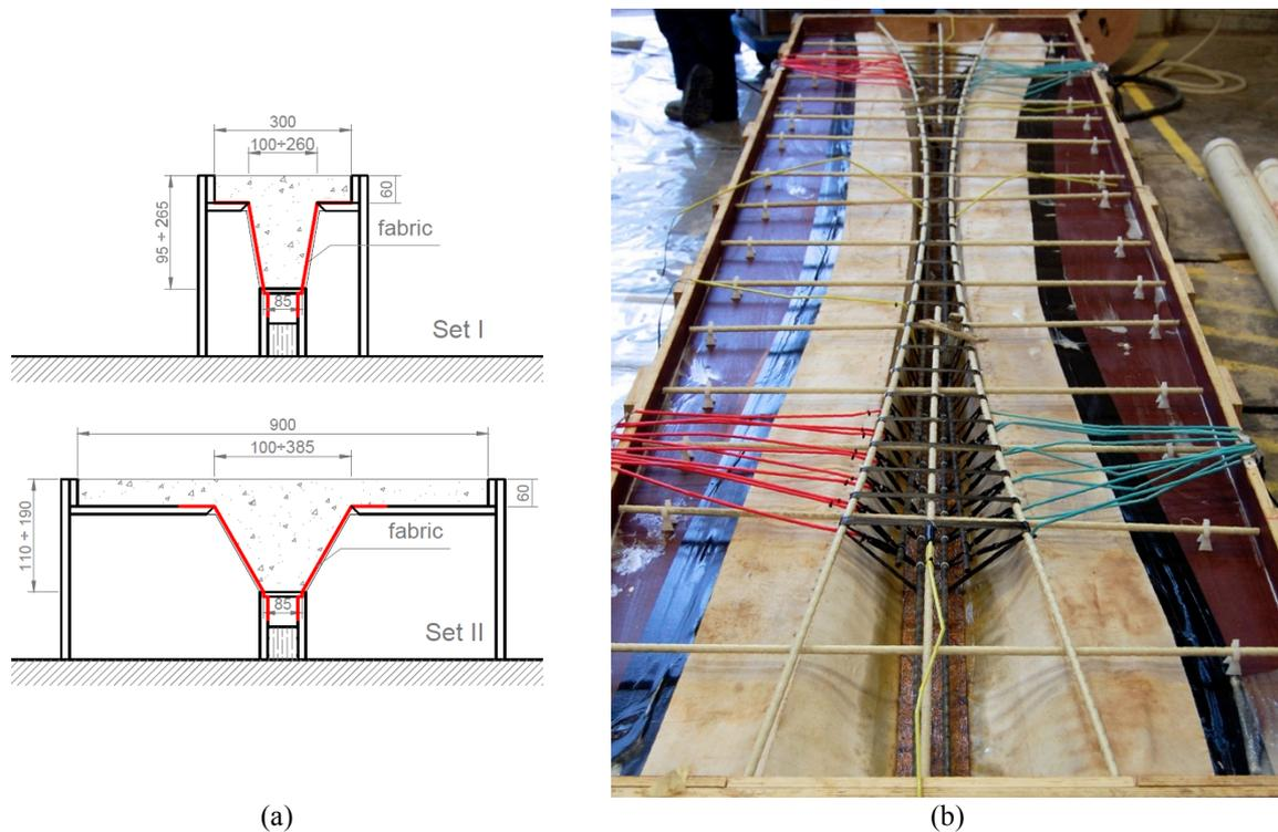
Figure 3: a) formworks cross-section diagram; b) instrumented W-FRP cages installed into the fabric formworks before concrete casting (beam II.2).
