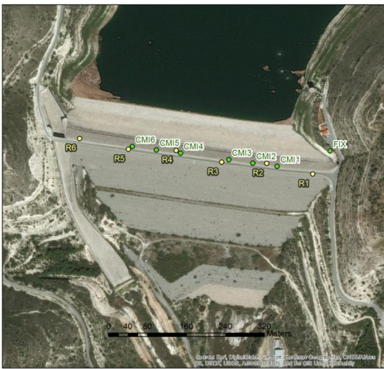
Figure 2: Instrumentation on the dam crest
