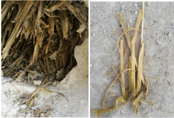
Figure 10. Opening of external render (left) and straw adjacent rendering layer (right) of low position of laid flat bale wall
