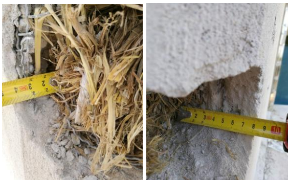
Figure 12. Straw conditions behind opening locations with thin rendering thickness (left) and thick rendering thickness (right)
