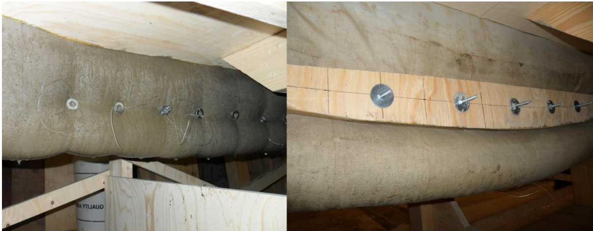
Figure 6 Internal restraints in fabric formwork using discrete ties or continuous web formers
