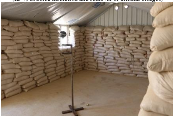
g) Thermal mass with internal sandbags (ID 6; Internal wall layer of 250 mm)
