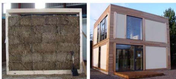
Figure 4 ModCell panel under construction in a 'flying factory' (left) and the completed prototype house at the University of Bath campus (right).
