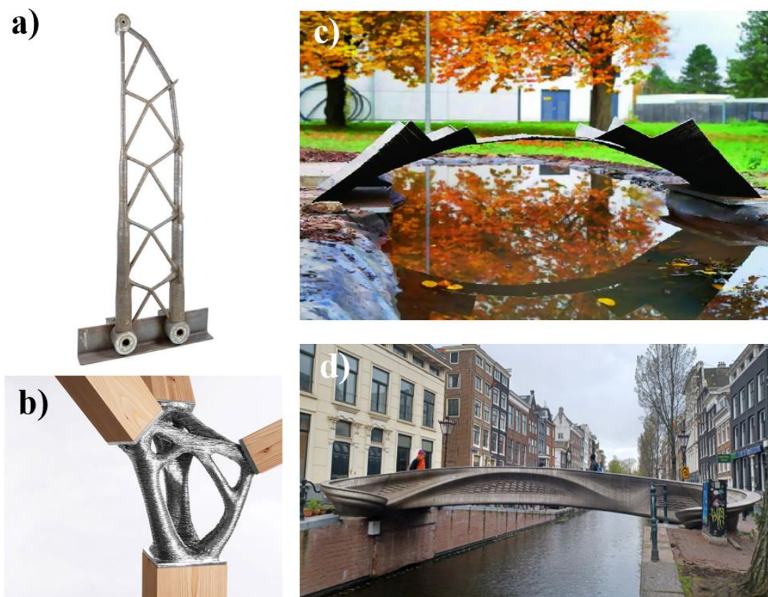
55 56 Figure 1: Successful examples illustrating the potential of WAAM in steel construction. a) 57 Truss structure with optimised member sizes [16]; b) connection of spatial shells [17]; c) the 58 bridge in Darmstadt [18]; d) MX3D bridge in Amsterdam (Photo taken by the authors). 59 Reprinting permission for these images has been obtained from the publishers[16]–[18].
