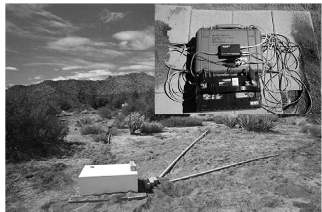
Figure 5. The ADU at Pinon Flat, California, with conduit running northeast and east to the two buried sensors; the inset shows the ADU, 12 V battery, and the fibre to Ethernet media converter.
