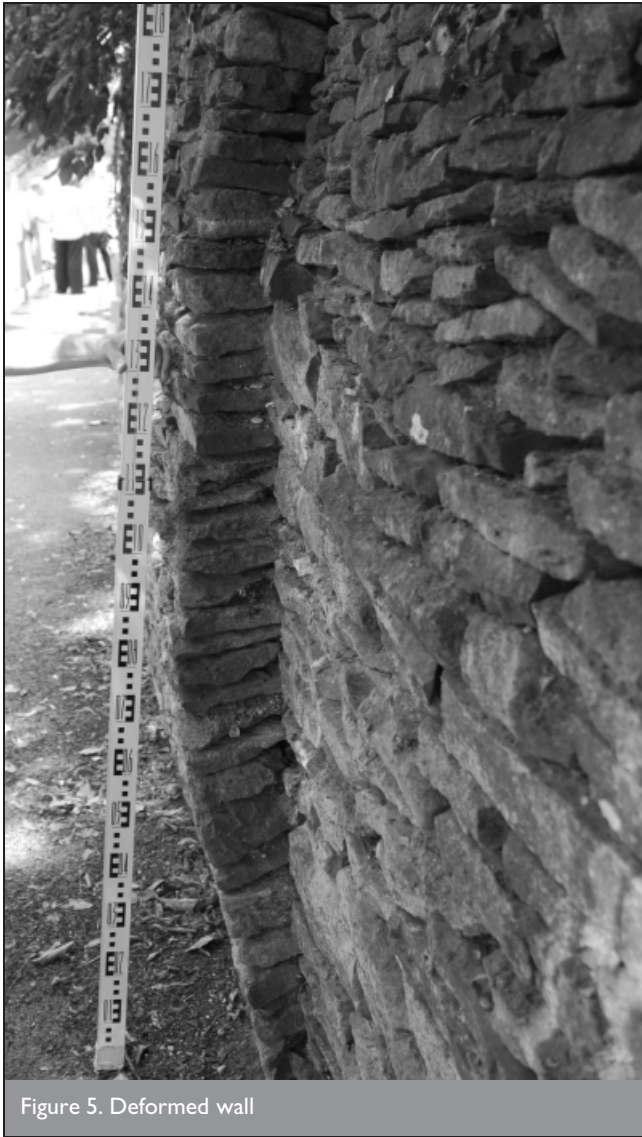
Figure 6. Section of typically bulged wall
