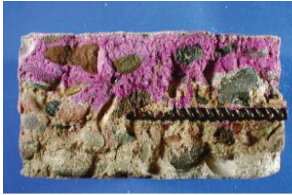
FIG. 1. Cross section of a reinforced concrete block. Pink indicates low pH, while colorless indicates a high one.
