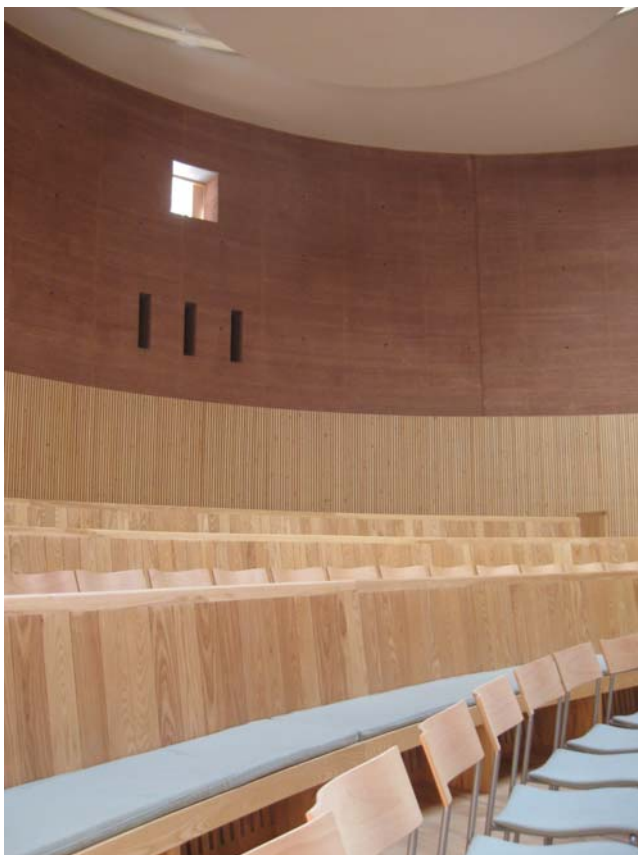
Figure 2. Sheppard Theatre, Centre for Alternative Technology, Wales: an example of a modern rammed earth structure
