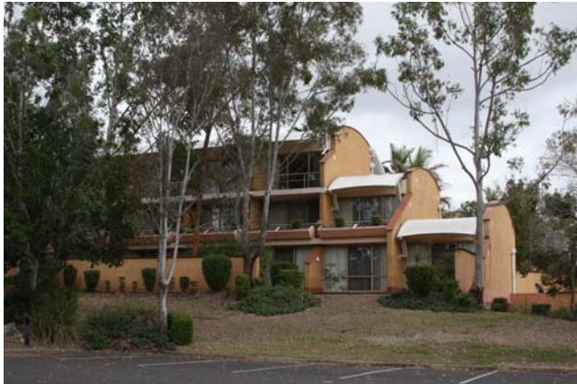
Figure 1. Kooralbyn Resort, Australia: an example of a modern rammed earth structure
